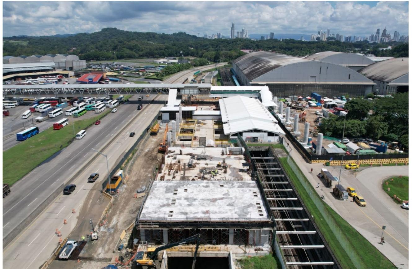
To cross the Canal, Metro de Panamá opted for a deep bored tunnel, abandoning the idea of using a shared deck on the Fourth Bridge. The result is one of the most technically demanding pieces of urban tunnelling in Central America: several kilometres of large-diameter tunnel at depth, in mixed ground, under a world-critical shipping lane.
