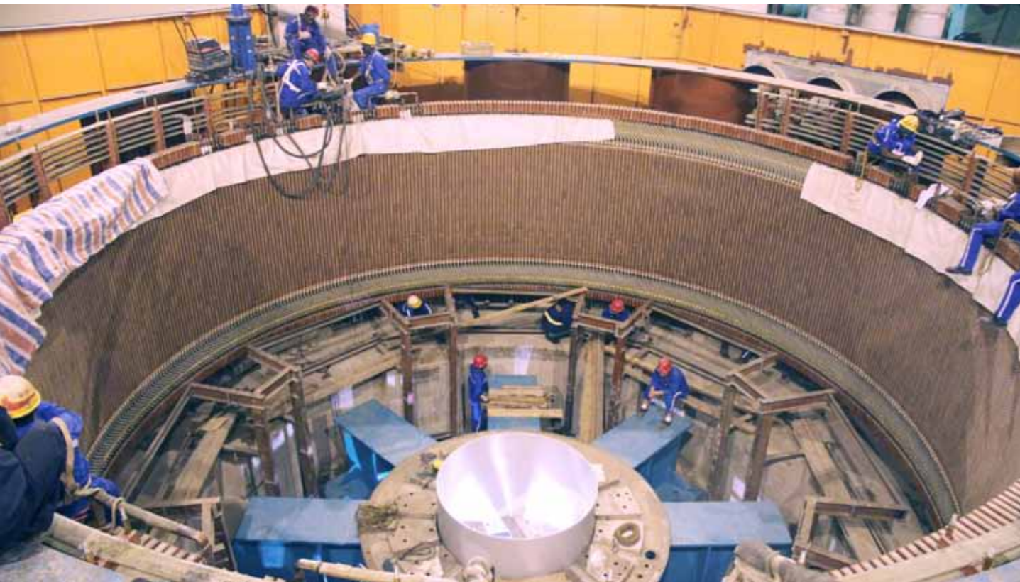
Work in progress at KNBE
