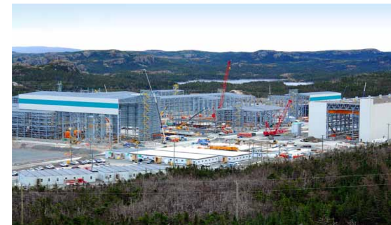
Main processing plant site
