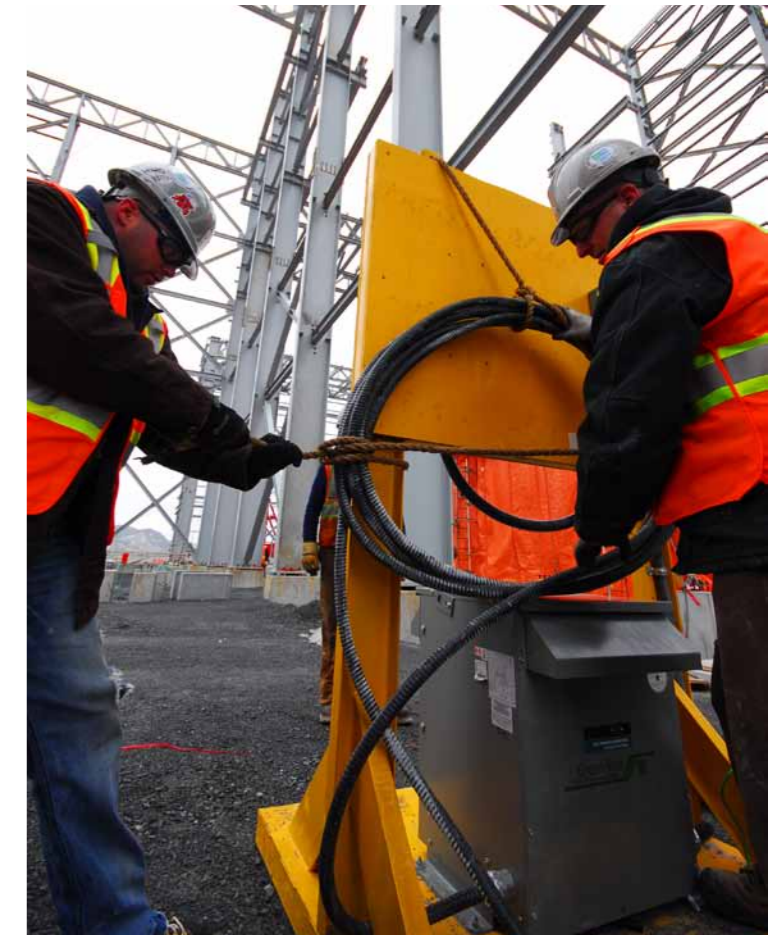
Workers installing temporary power
