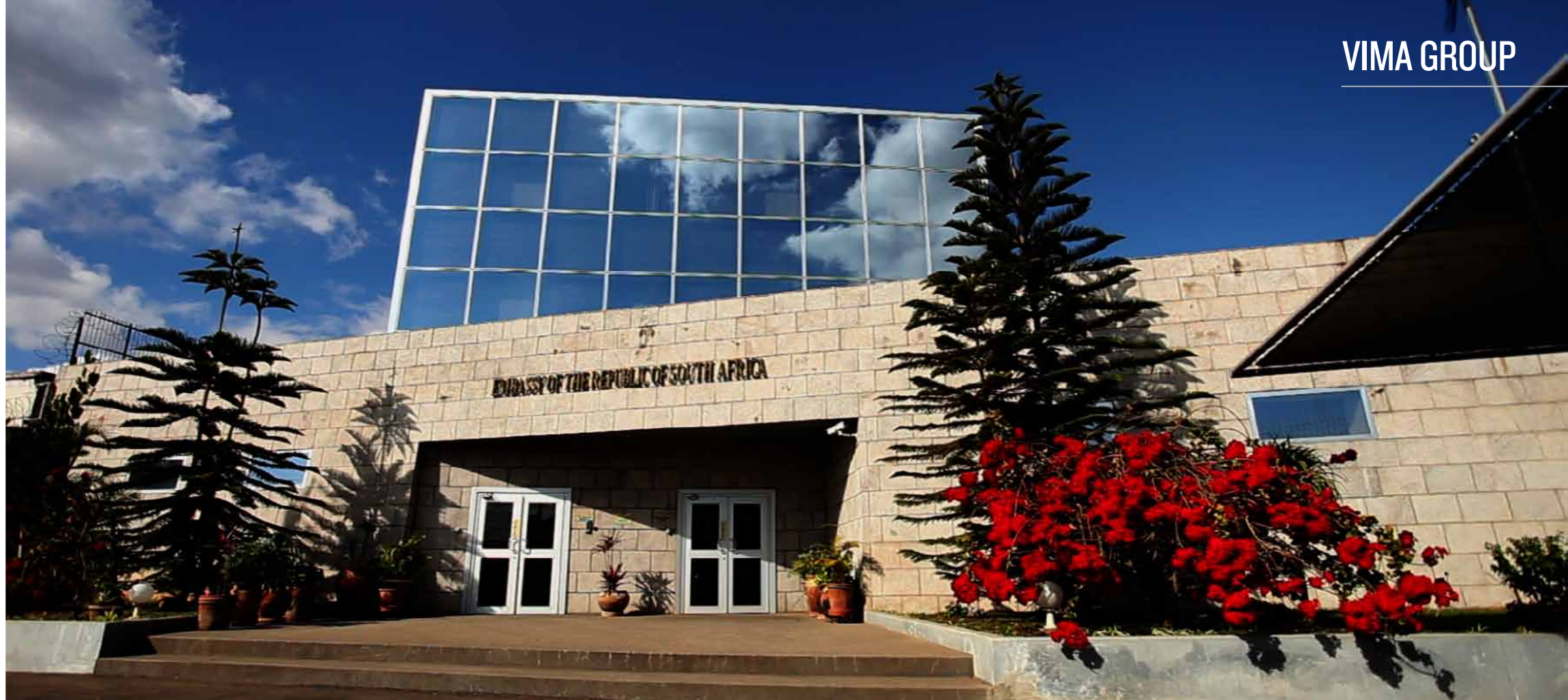
VIMA companies undertook the real estate services, procurement and construction for South Africa's new Embassy building in Madagascar
