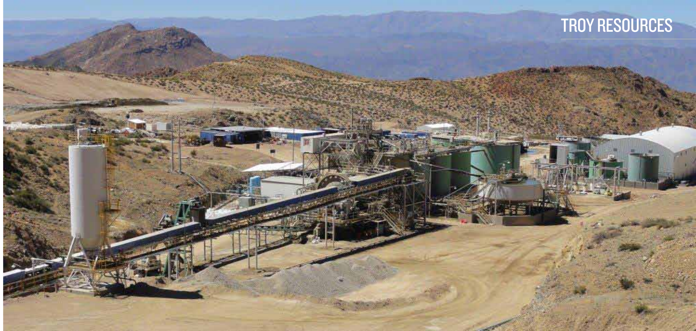
Casposo processing facility
