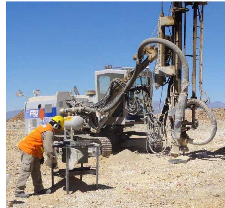
Production drilling – Kamila open cut
