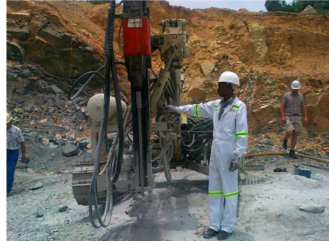
Testing of S140 on site
