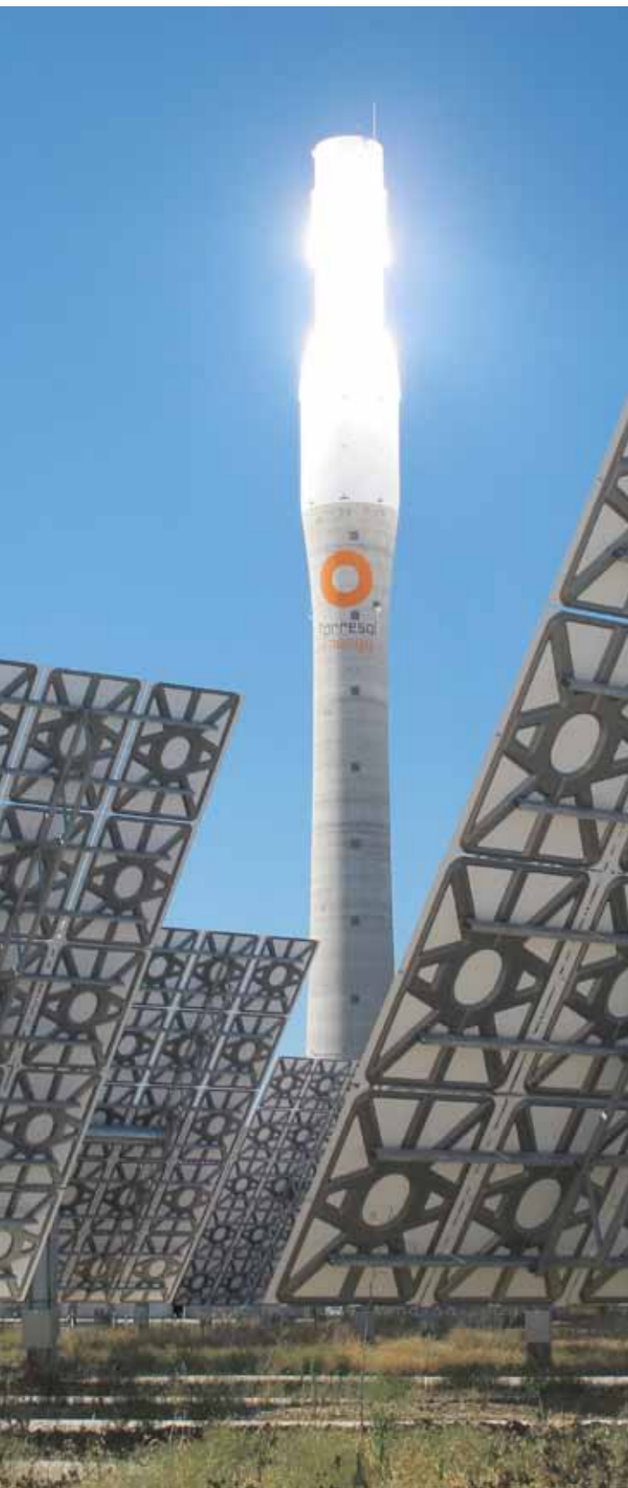
Tower and heliostats
