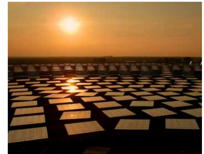
Heliostat field at dusk
