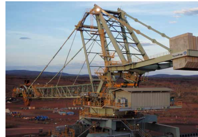
Iron ore reclaimer at a mine near Newman, WA
