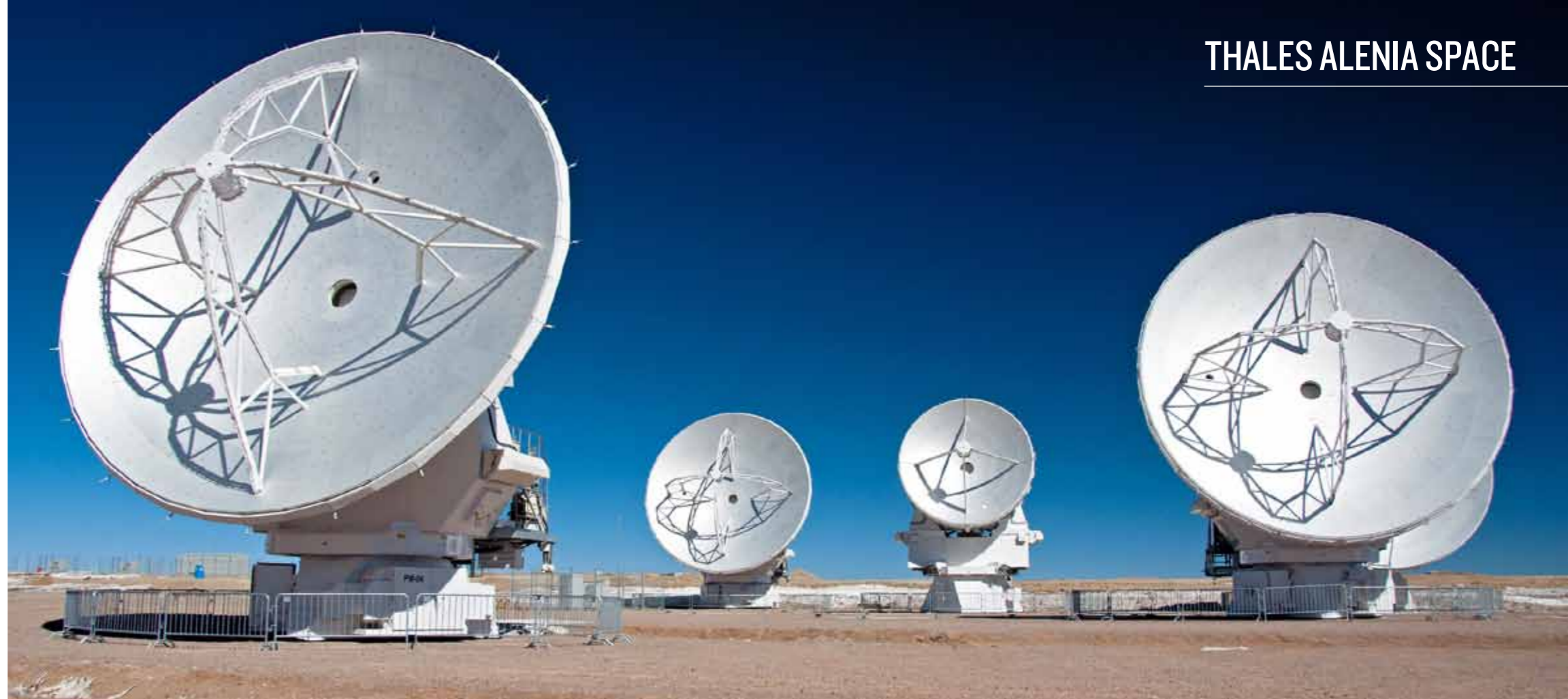
Antennas onsite and assembled
