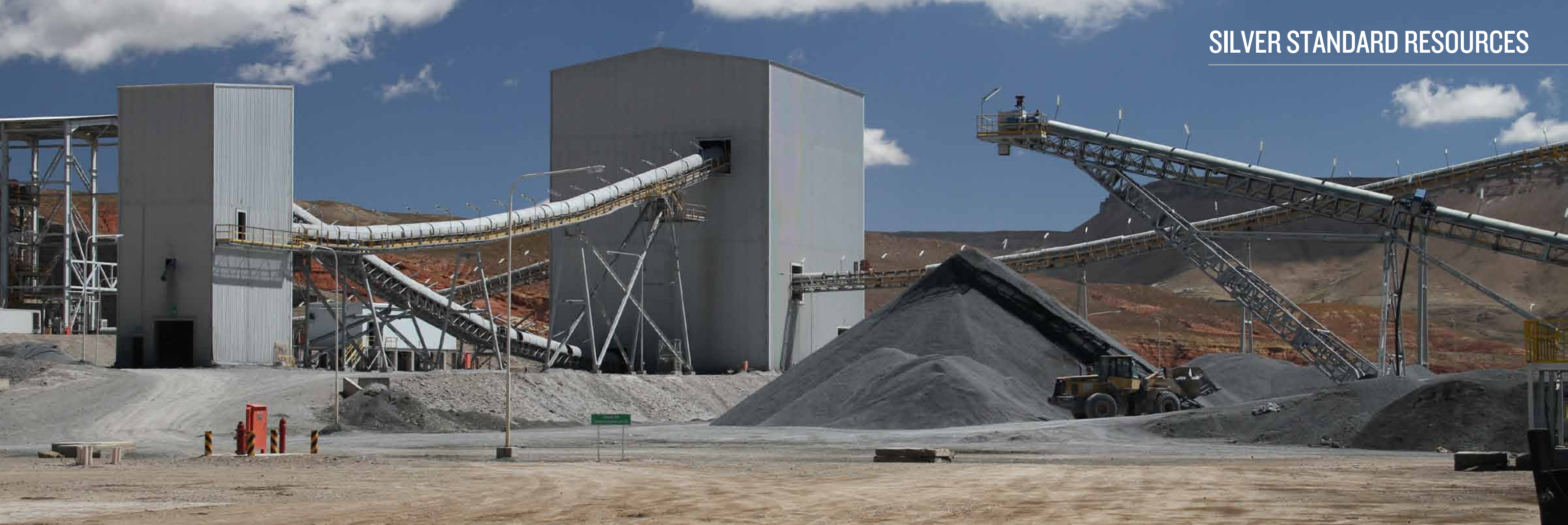
The crushing plant and the coarse ore stock pile at Pirquitas Mine
