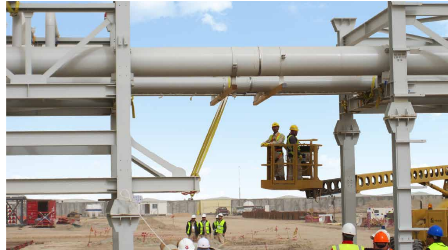
Perfect fit of two pipe rack modules at site
