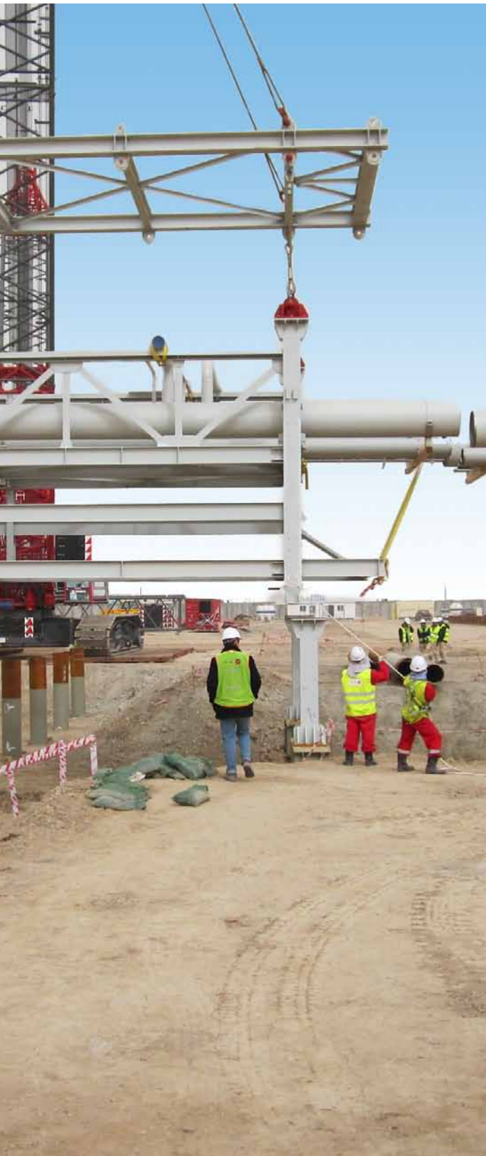
Erection of second pipe rack module
