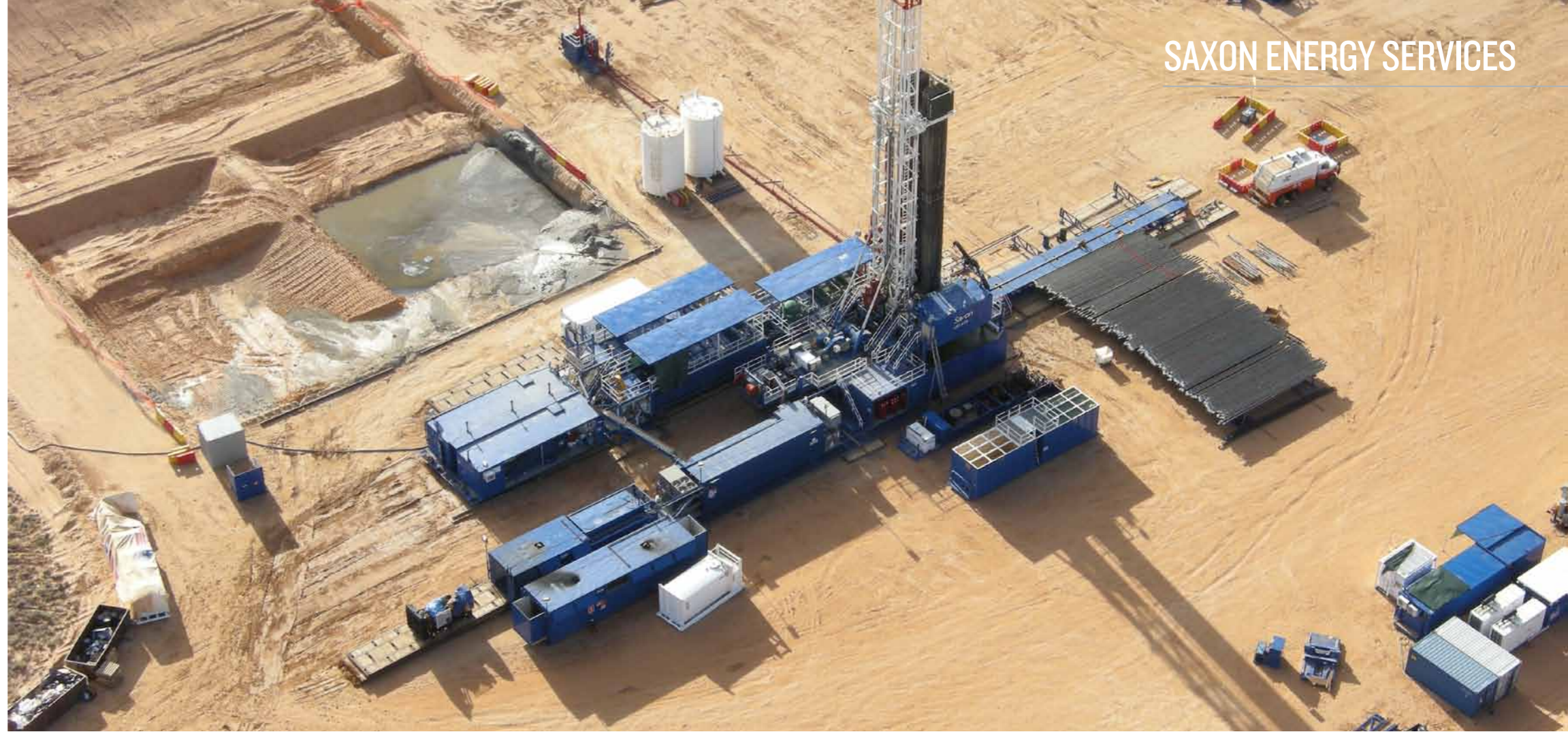
Aerial view of Saxon rig
