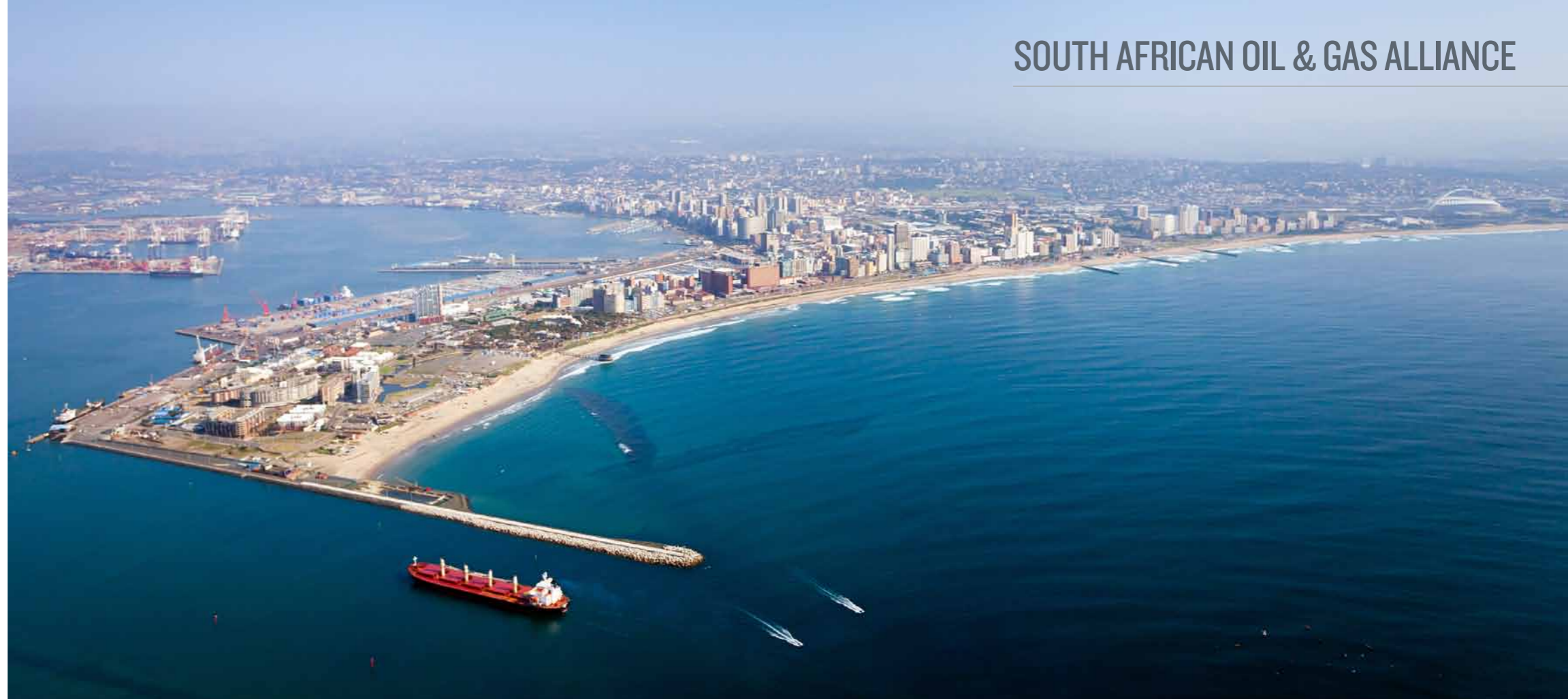
Established road, rail, sea and air routes make South Africa makes an ideal logistics base
