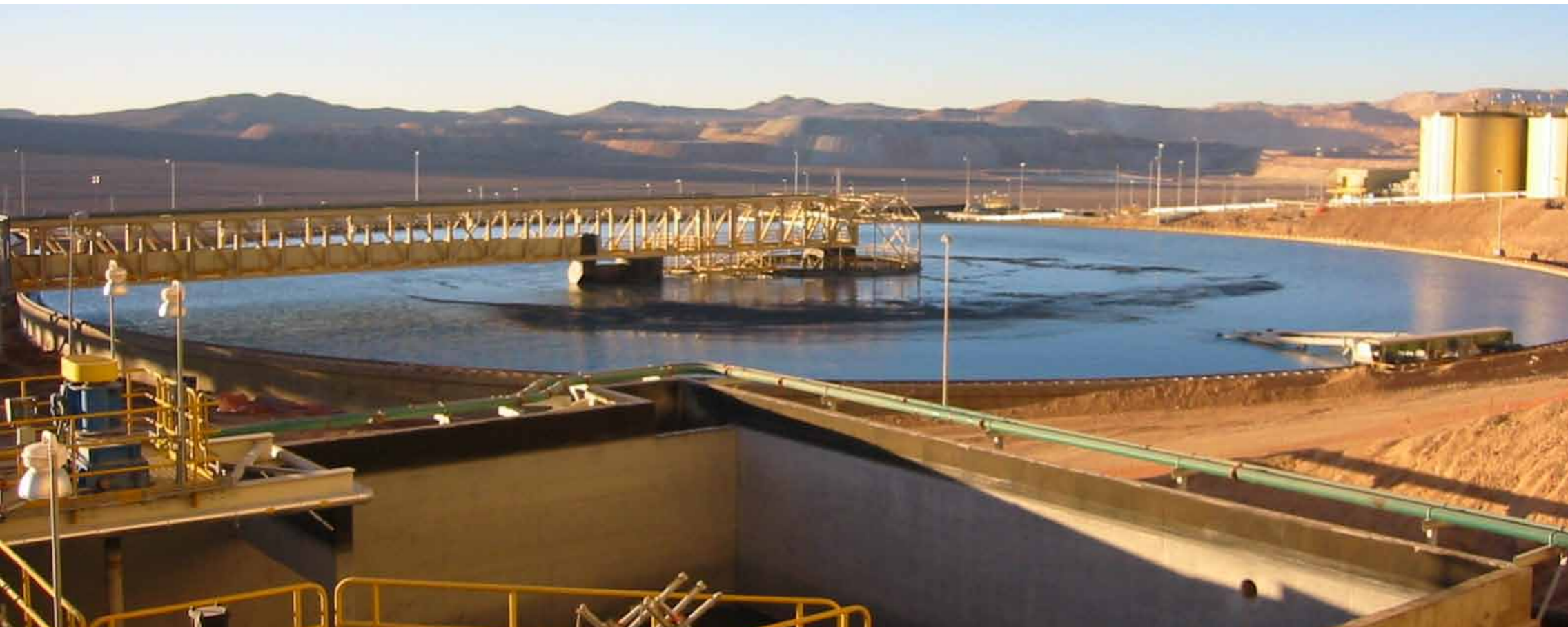
Copper thickener in the Atacama Desert, Chile
