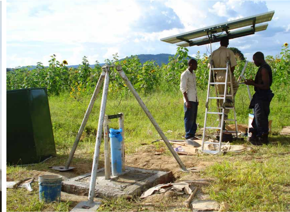
Village solar water pump installation
