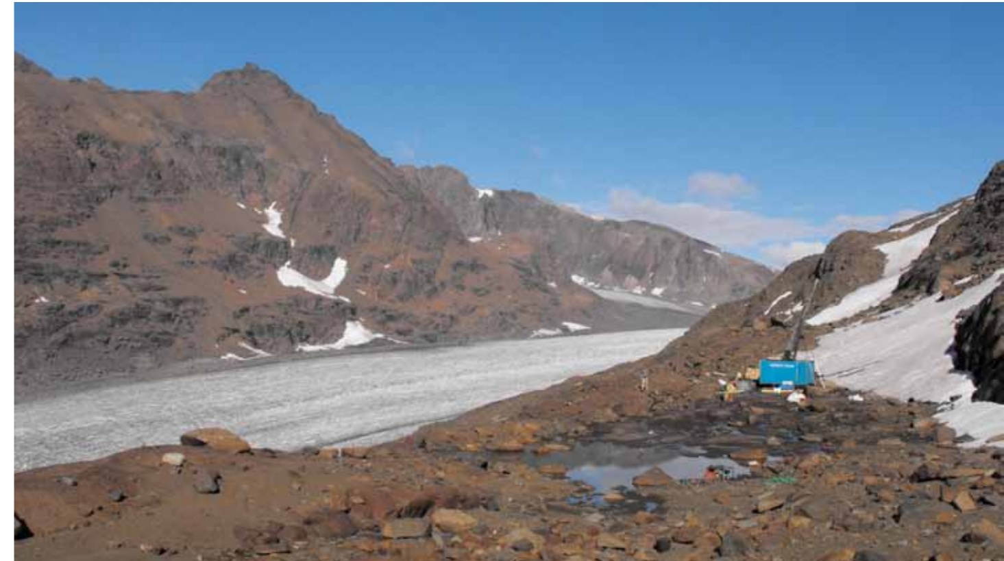
Drill Rig operating at Skaergaard Project, East Greenland
