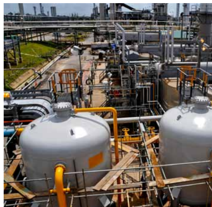
Overlooking the water treatment plant
