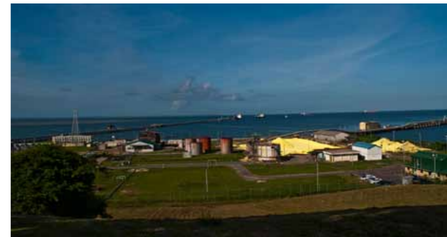
Port facilities at Pointe-à-Pierre
