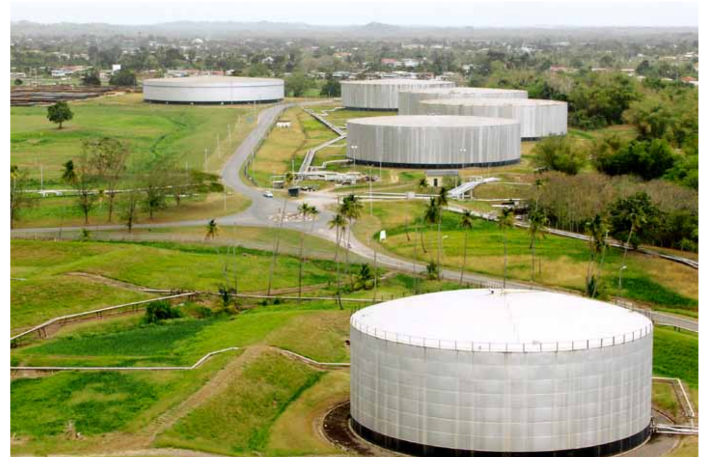
Tank farm in harmony with the landscape
