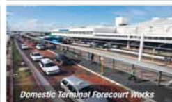
Domestic Terminal Forecourt Works
