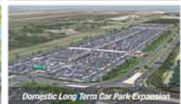
Domestic Long Term Car Park Expansion
