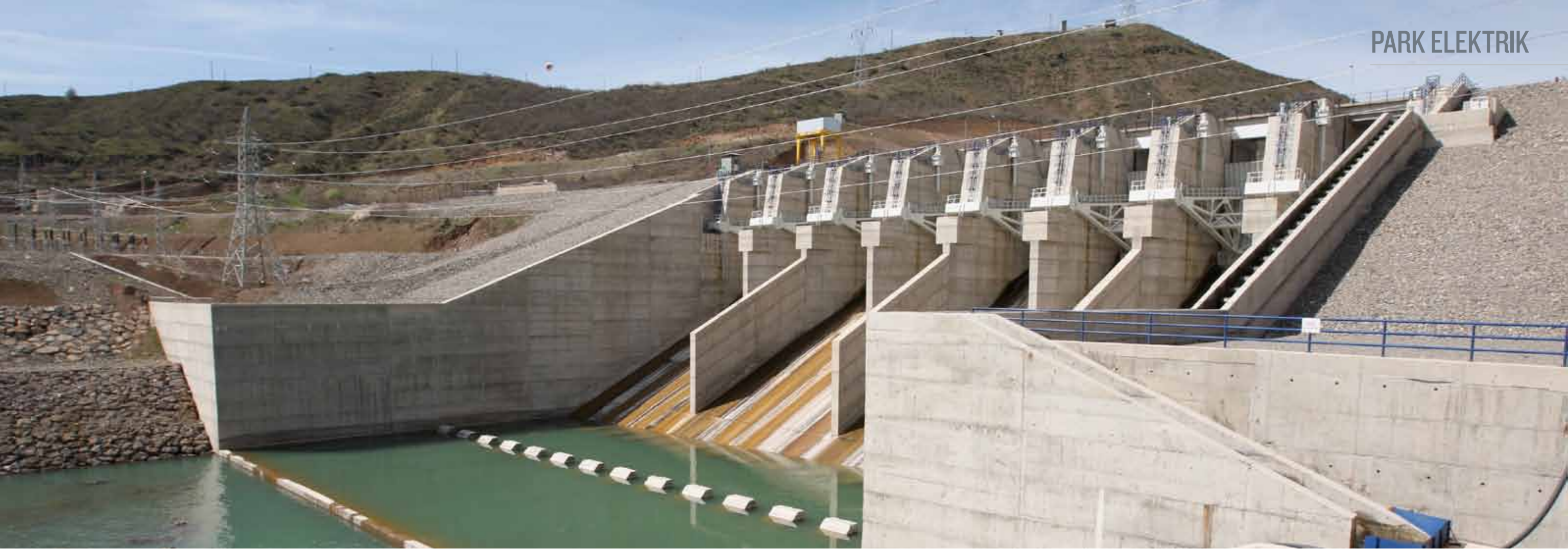
Hydro-electric power station in Turkey
