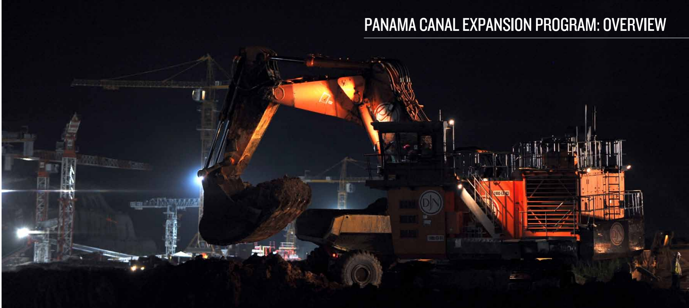
Construction continues day and night at the new Atlantic Lock site
