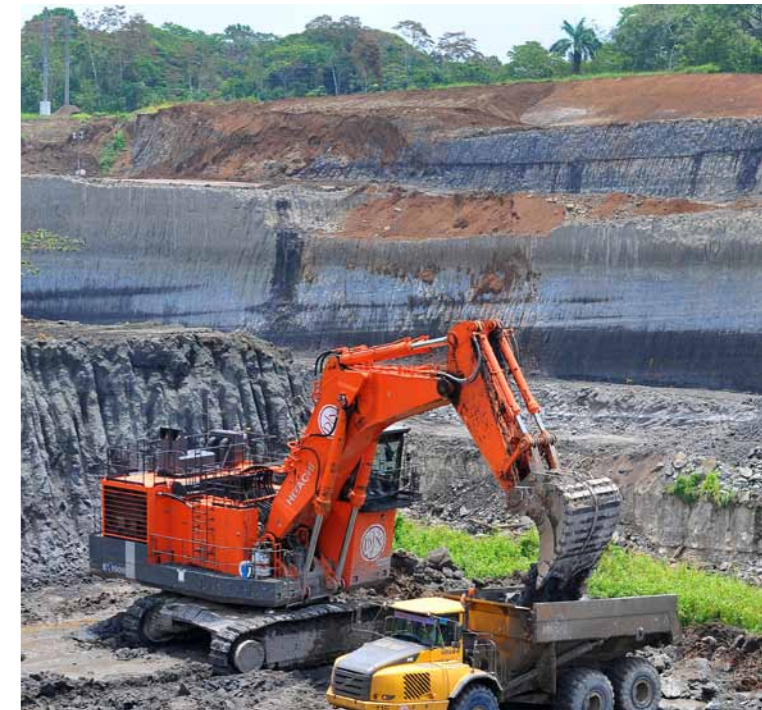
Excavation has been split into four contracts
