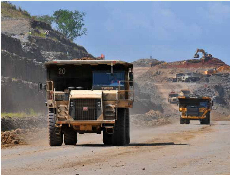
Removing excavated material is an ongoing process
