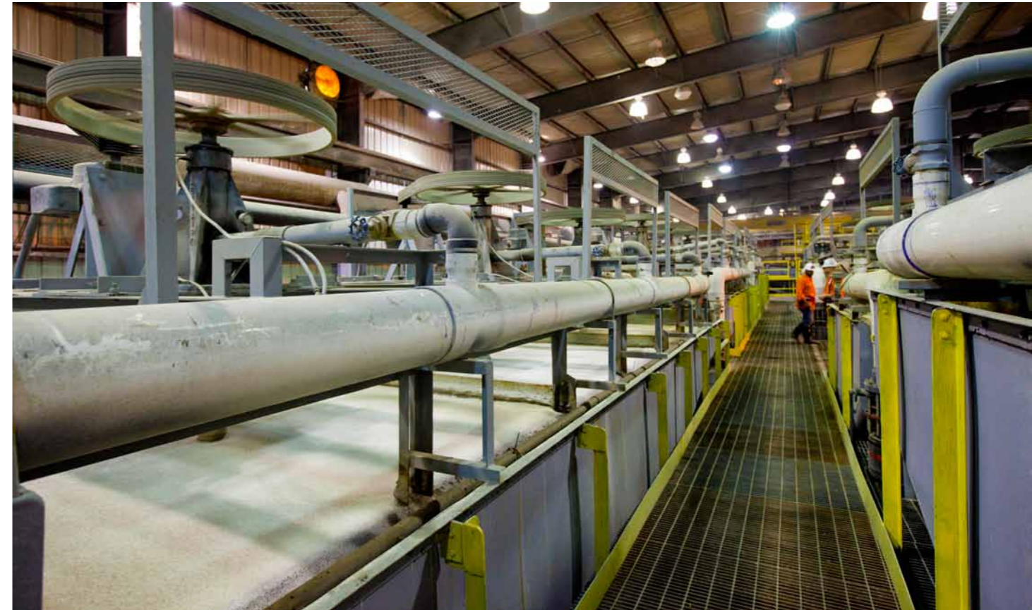
Inside the Gordonsville mill
