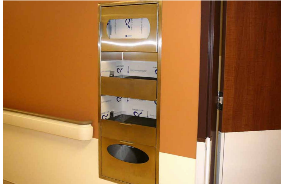
Supply storage for gowns, gloves and masks were built into the walls outside of inpatient rooms to avoid clutter being created in hallways
