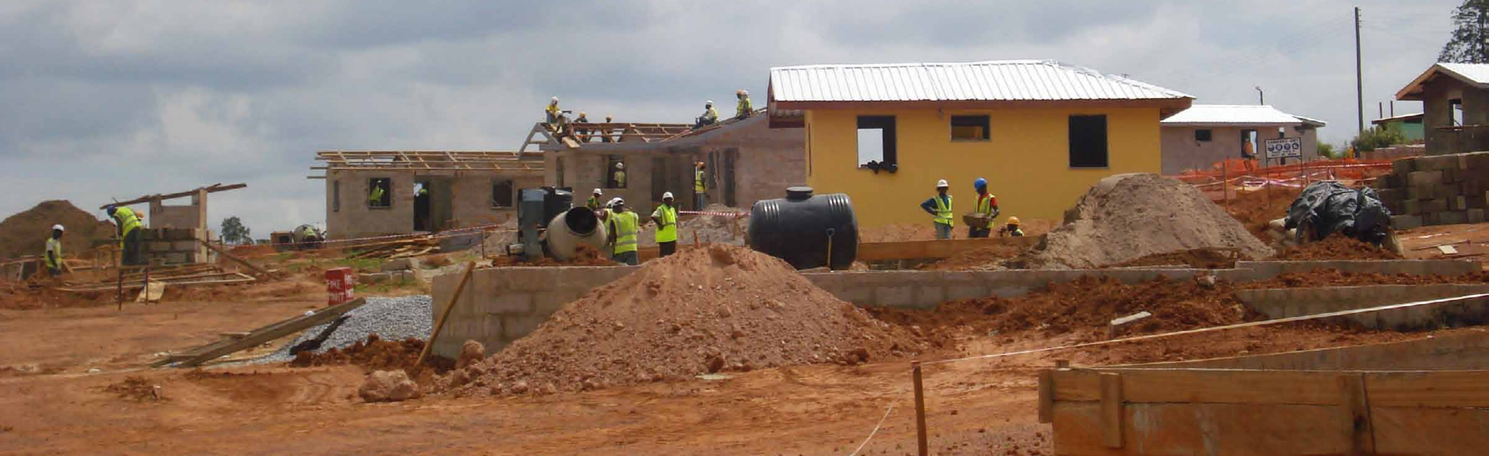
Ahafo local contractor building resettlement housing
