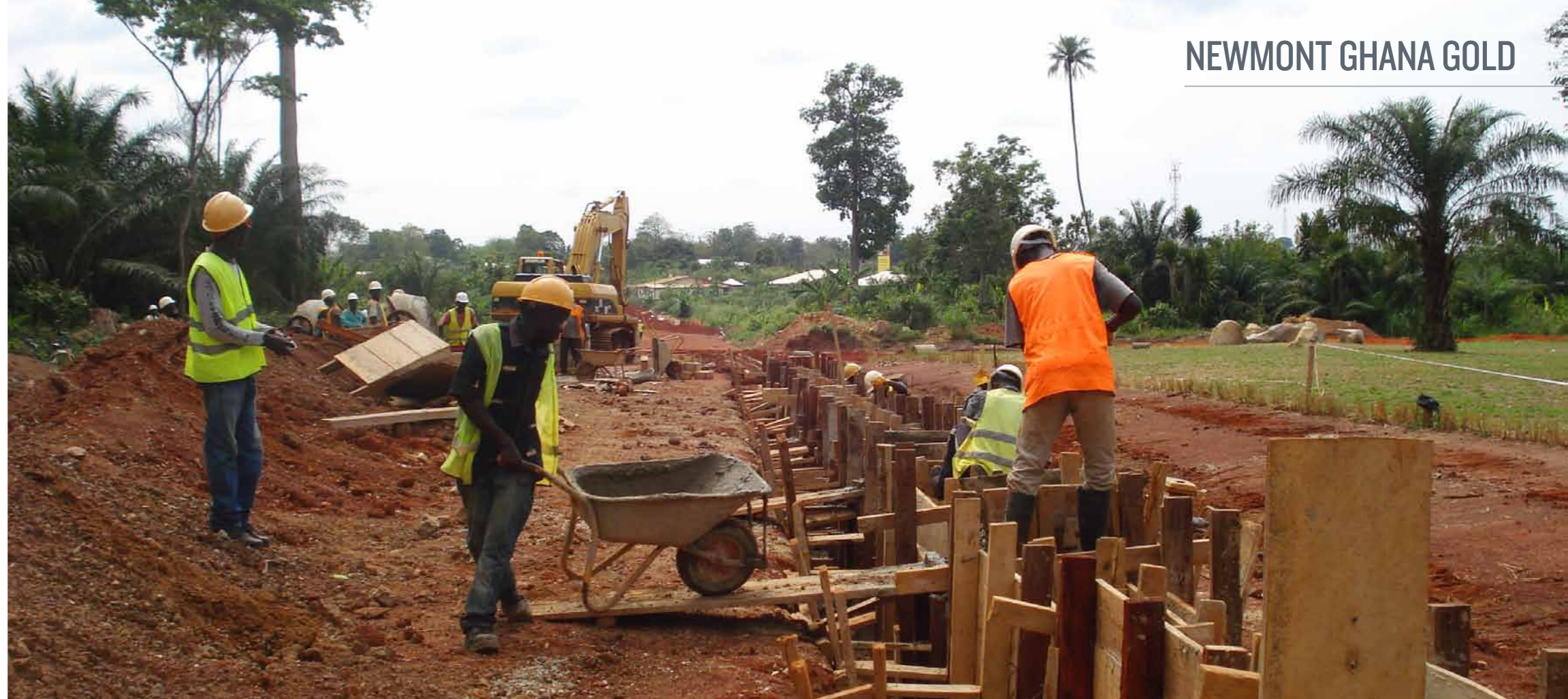
Ahafo local business constructing drainage system at resettlement site
