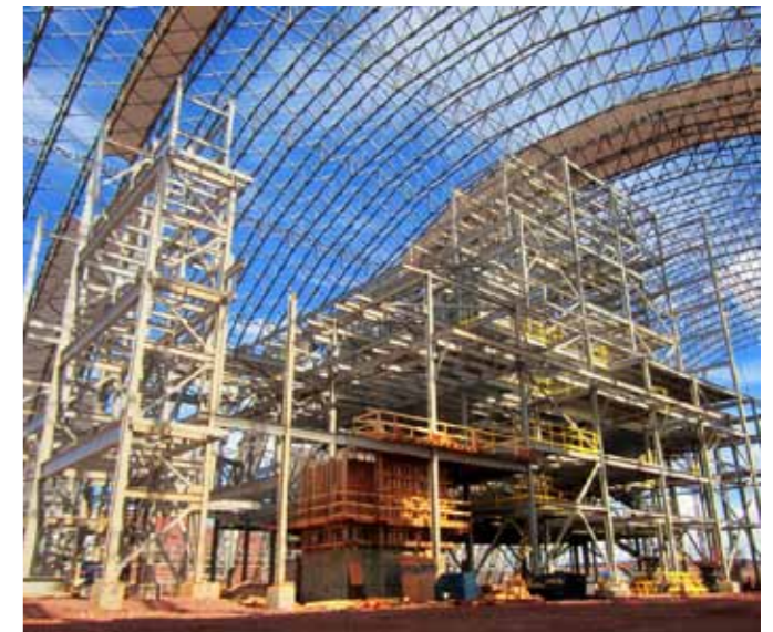
Erection of the process plant building
