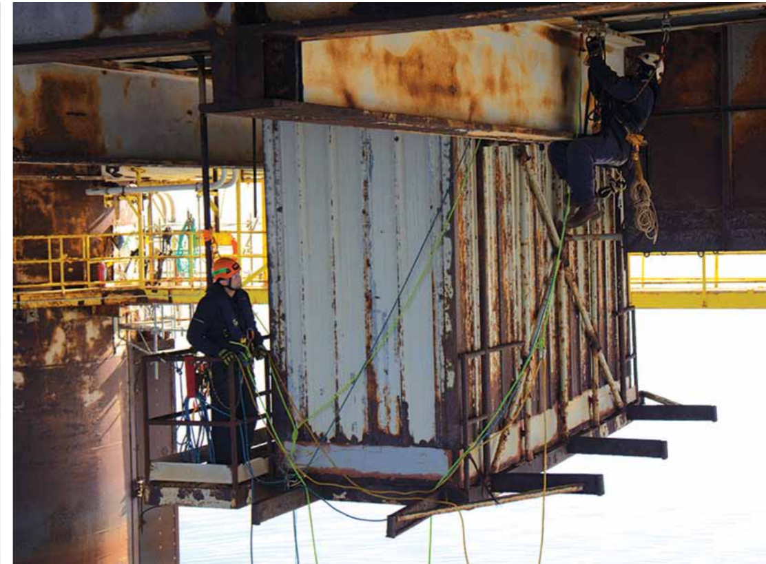
Under-deck inspection using rope access
