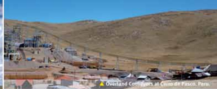
▲ Overland Conveyors at Cerro de Pasco, Peru.
