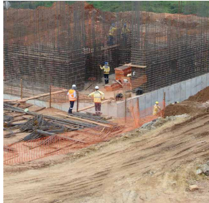
Construction in progress
