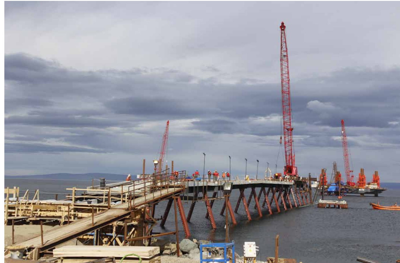
Construction of the new port
