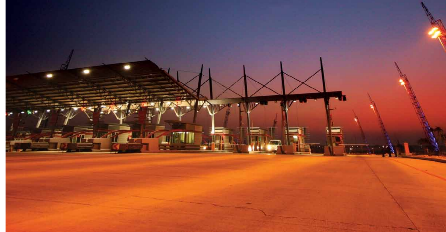
Diamond Hill toll plaza on N4
