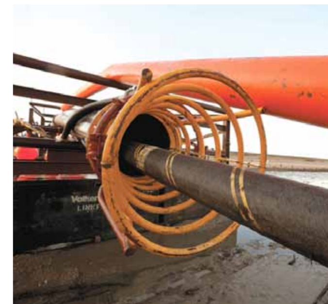
Installing array cables
