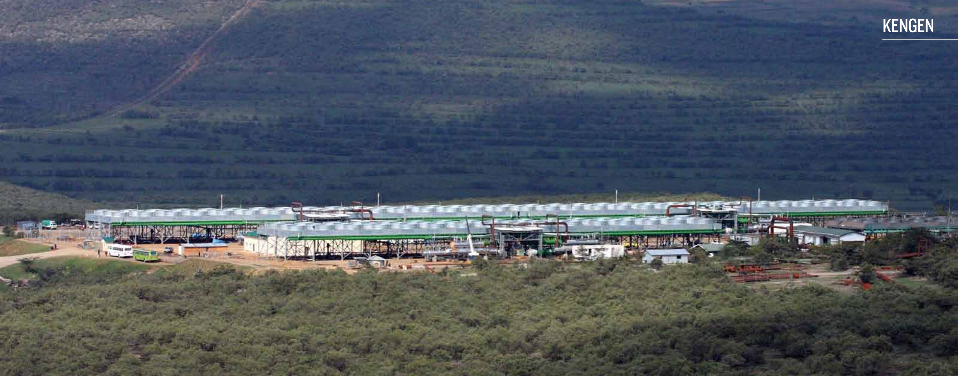
The Olkaria III power plant
