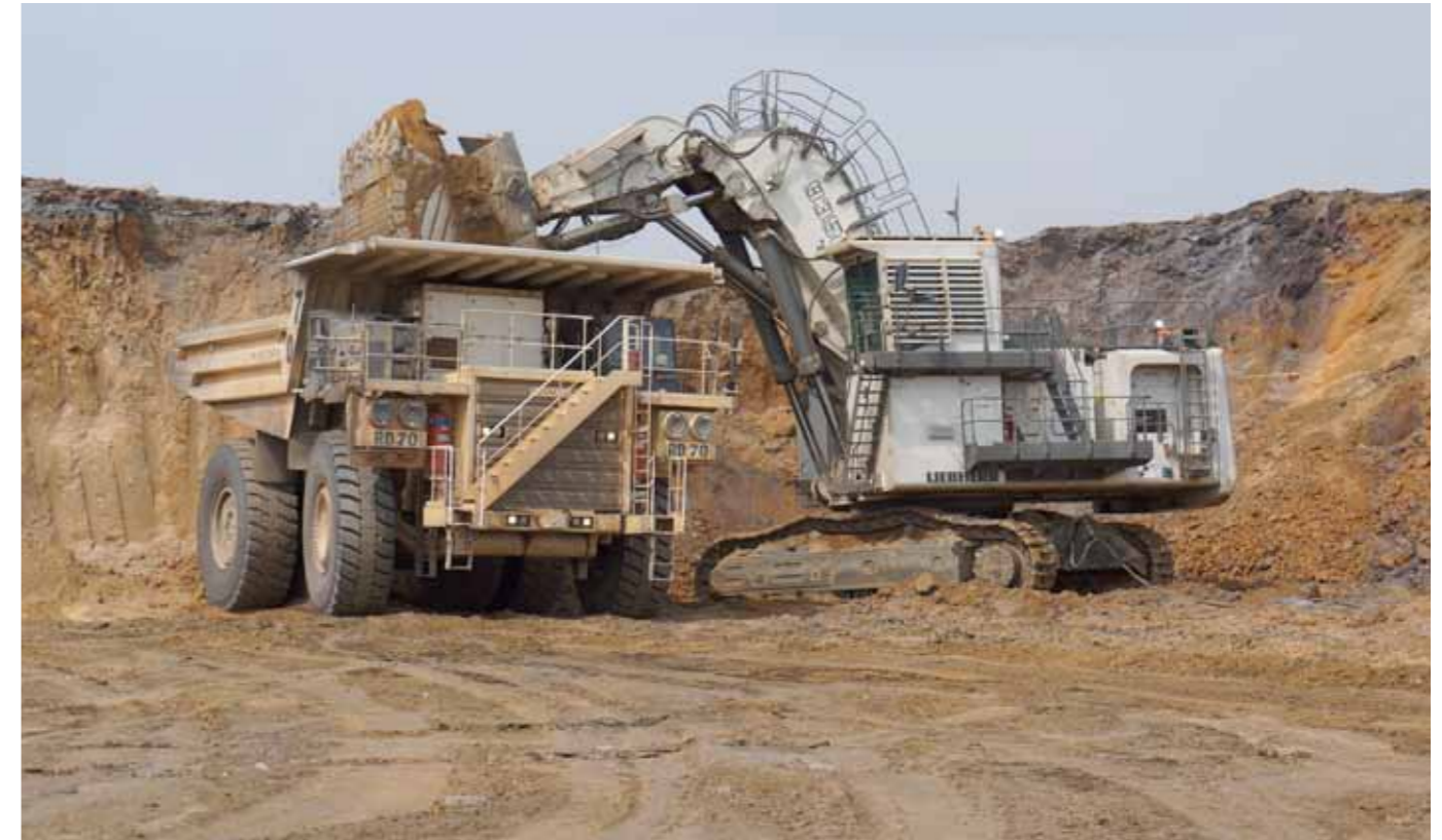
Excavation taking place
