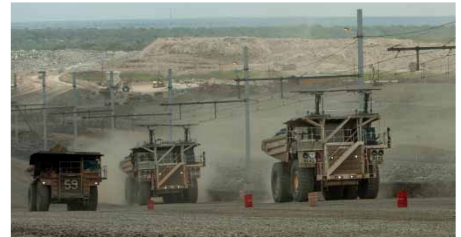
The Kansanshi mine is aiming to become as self sufficient as possible
