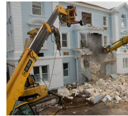
Old hospital demolition (March 2011)
