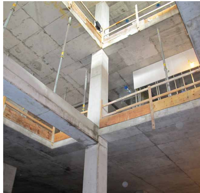
Looking up through the new hospital facility construction
