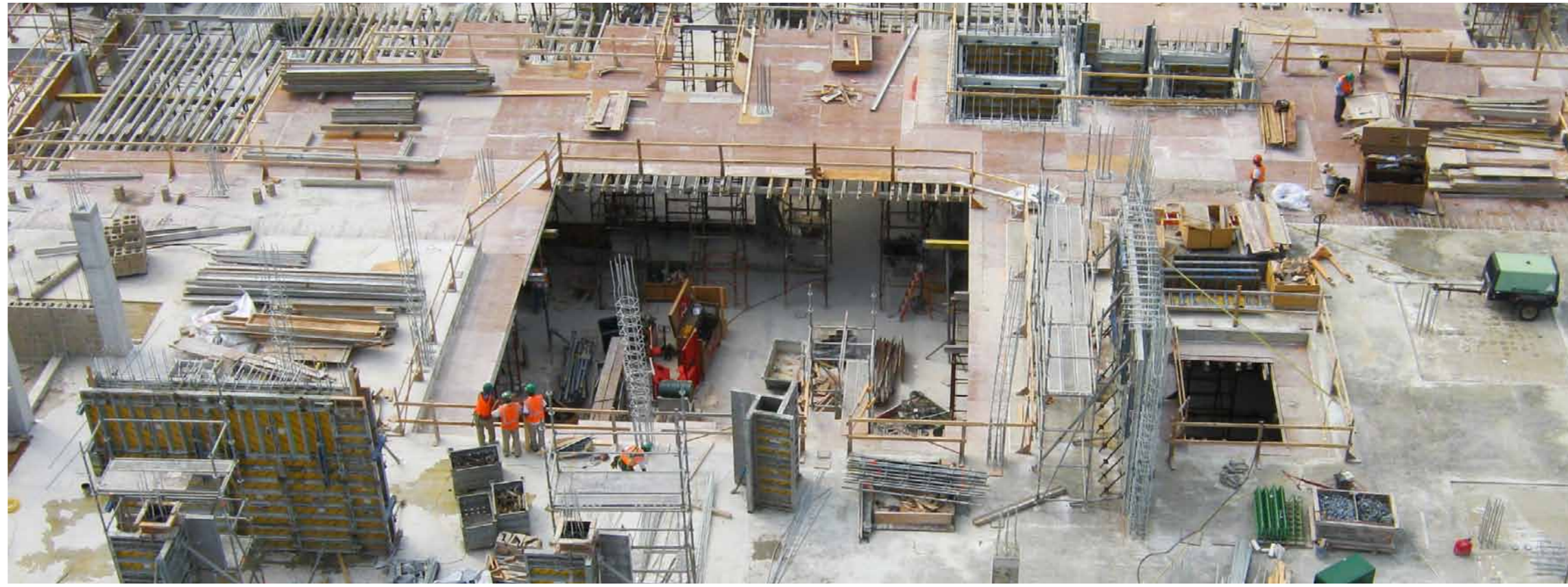
Aerial view of the new hospital facility under construction in June 2012
