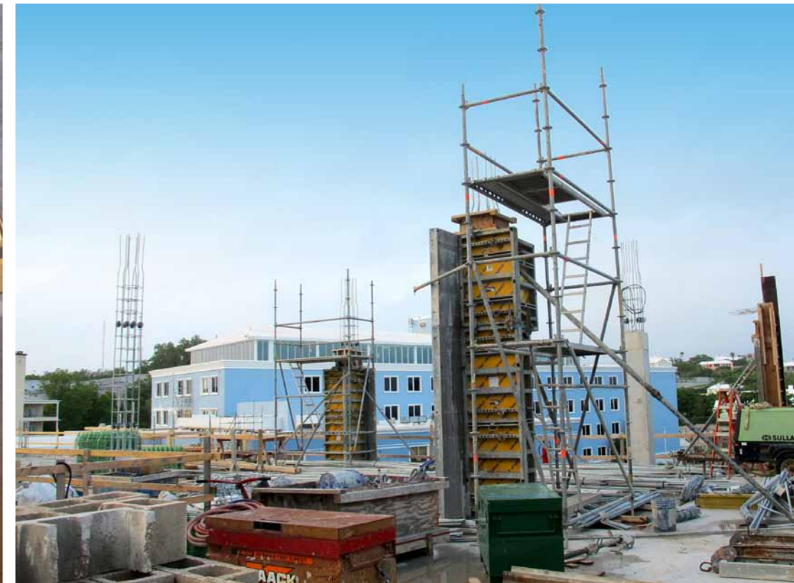
Construction had reached the third floor in July 2012
