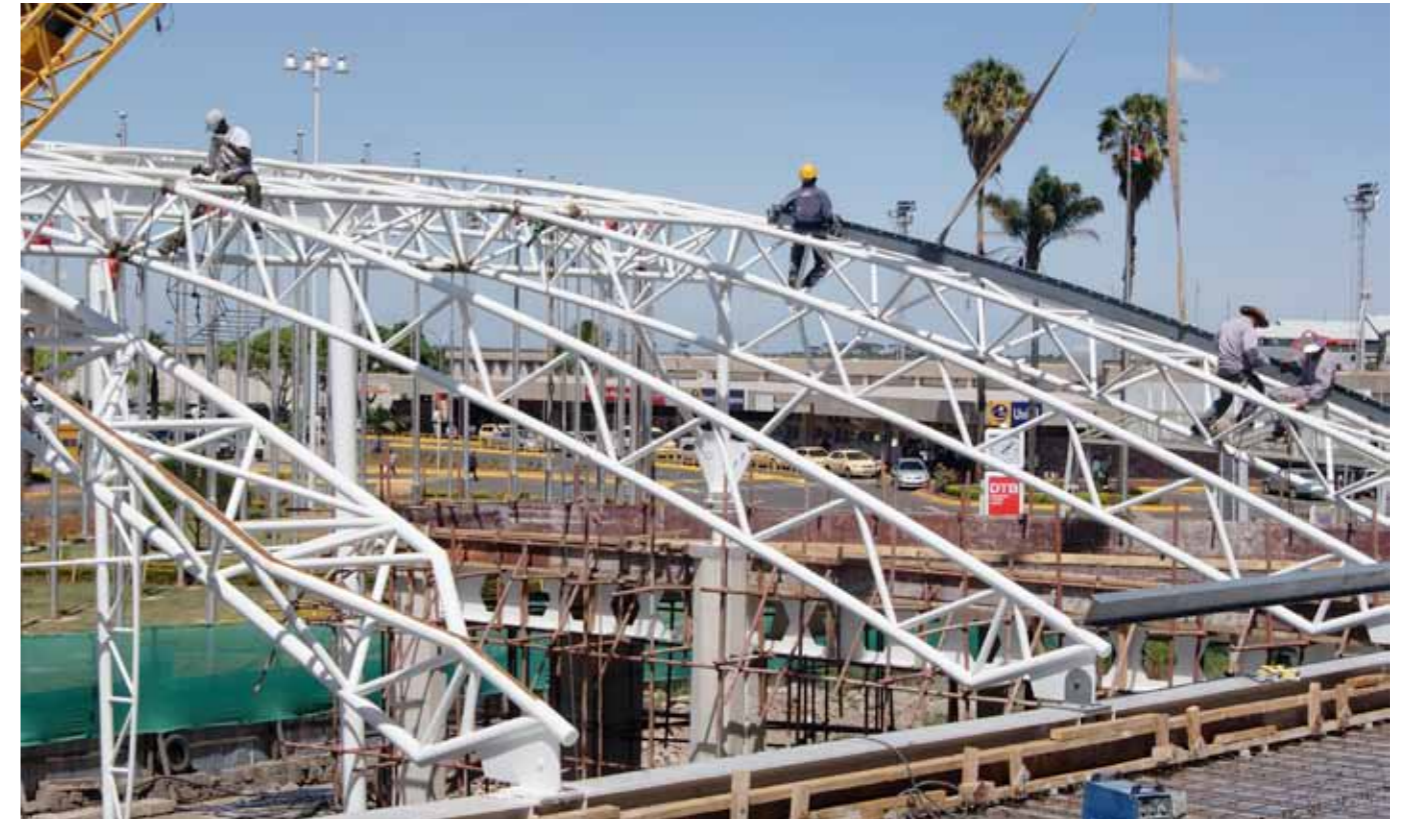
Construction taking place
