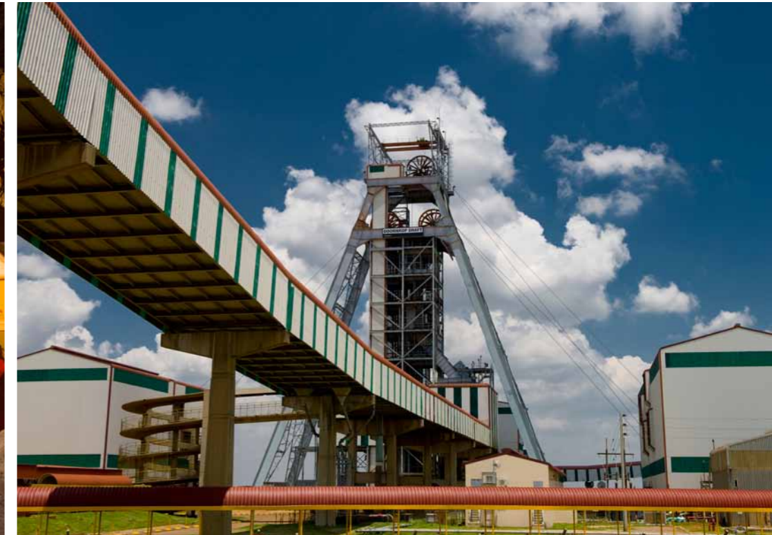
Headgear of Doornkop in Gauteng, South Africa
