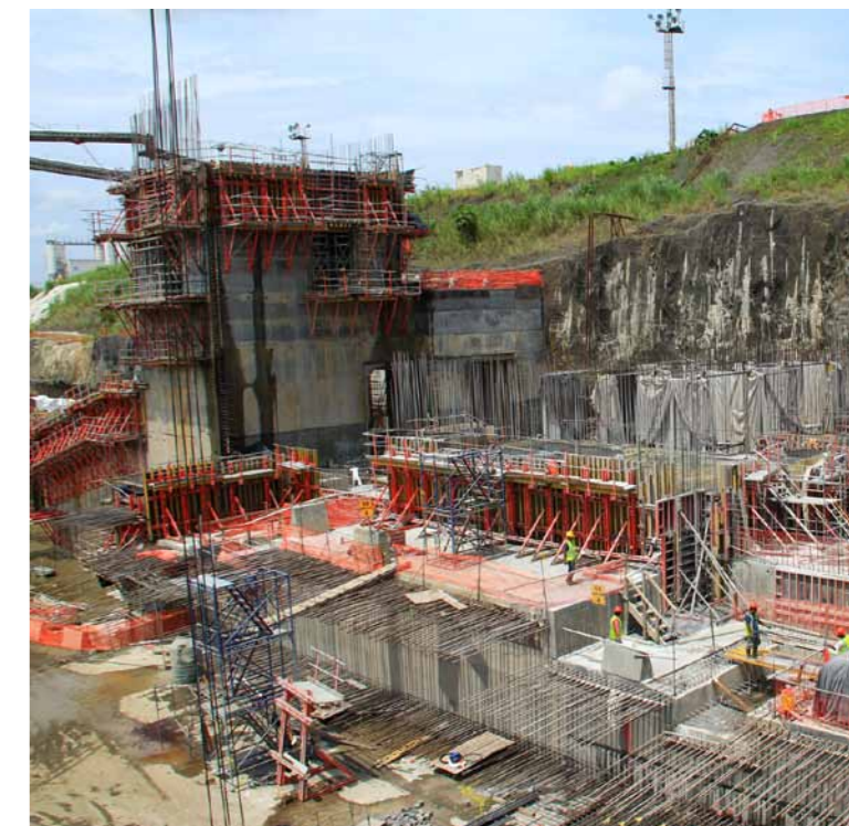
Construction under way on the Pacific site
