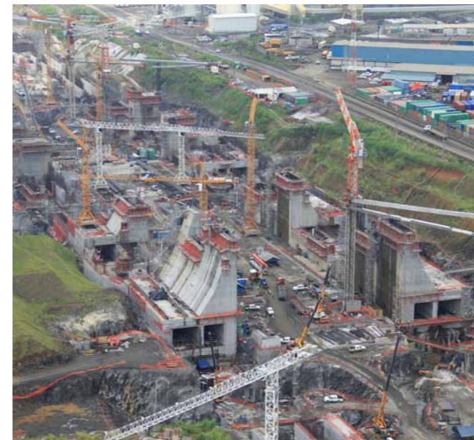
Upper chamber construction
