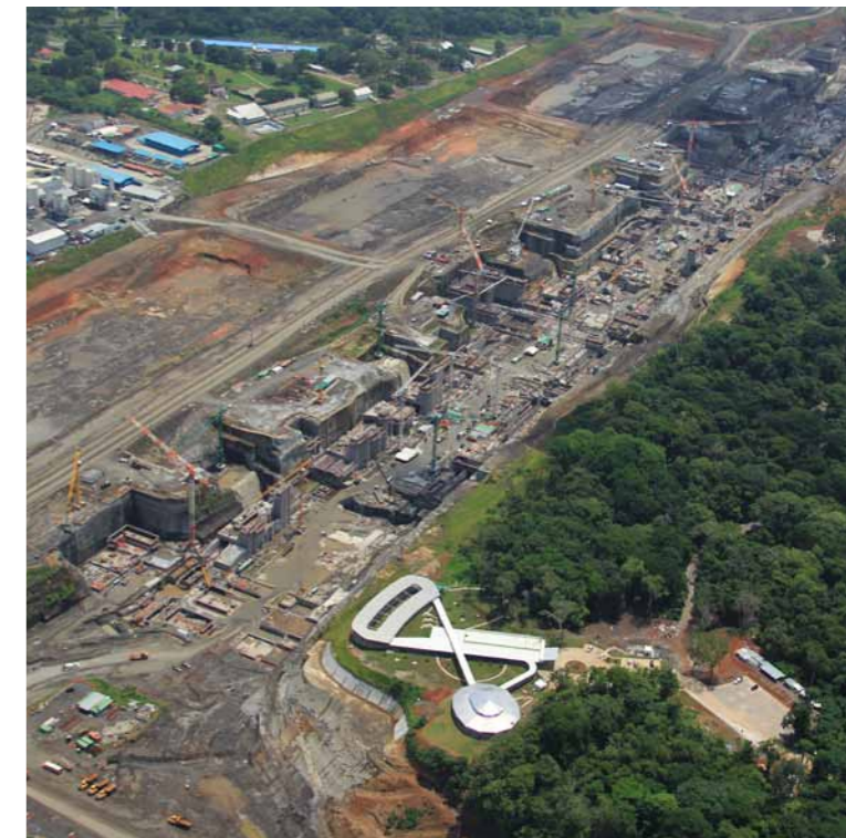
Atlantic lock construction
