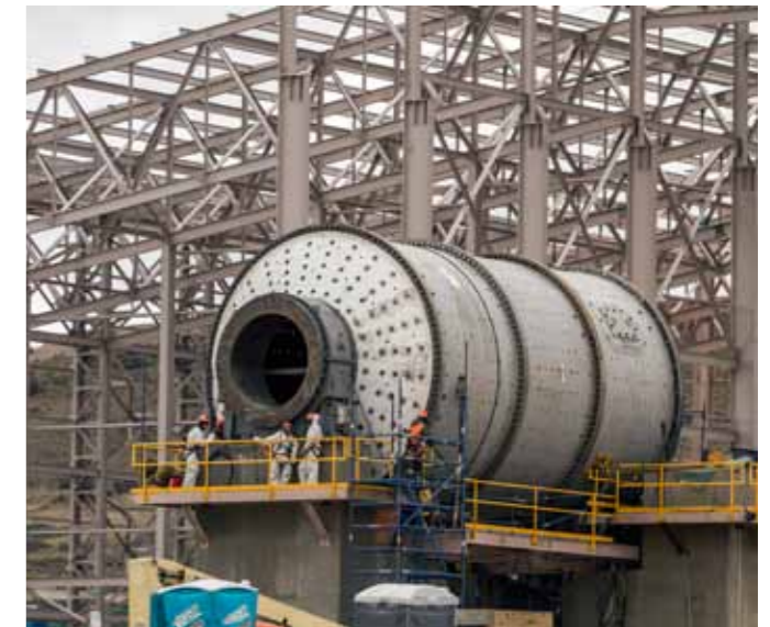
Plant construction – Vein Zone area
