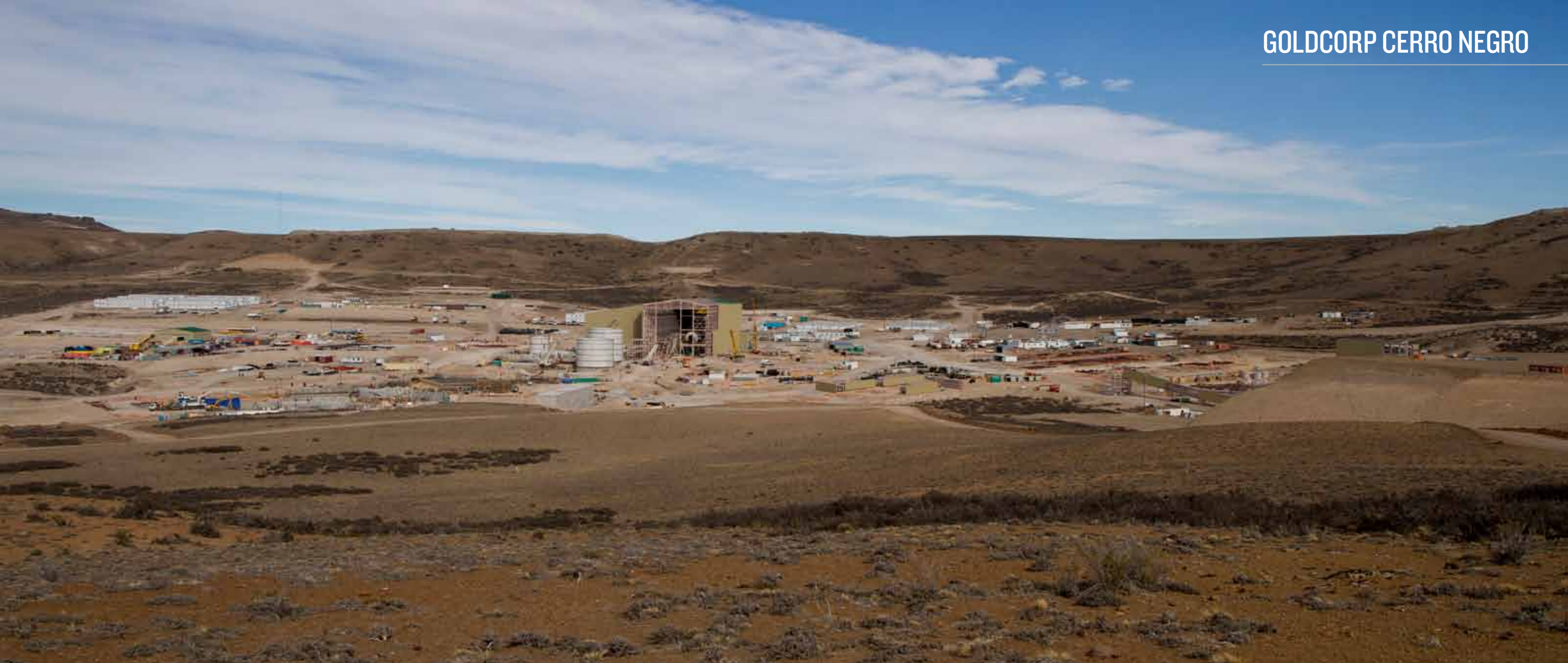
Panoramic view of plant construction in Vein Zone area
