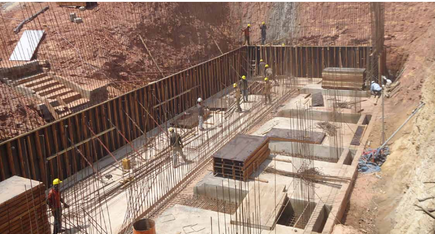
Works in progress on sub-structure for filter station at Mampong
