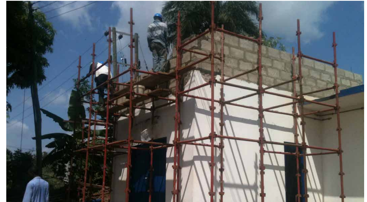
Booster station under construction in Kumasi
