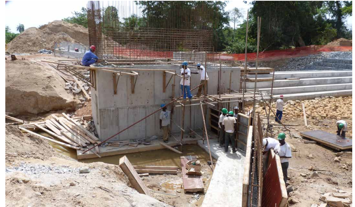
A weir and an intake under construction at Essakyir
