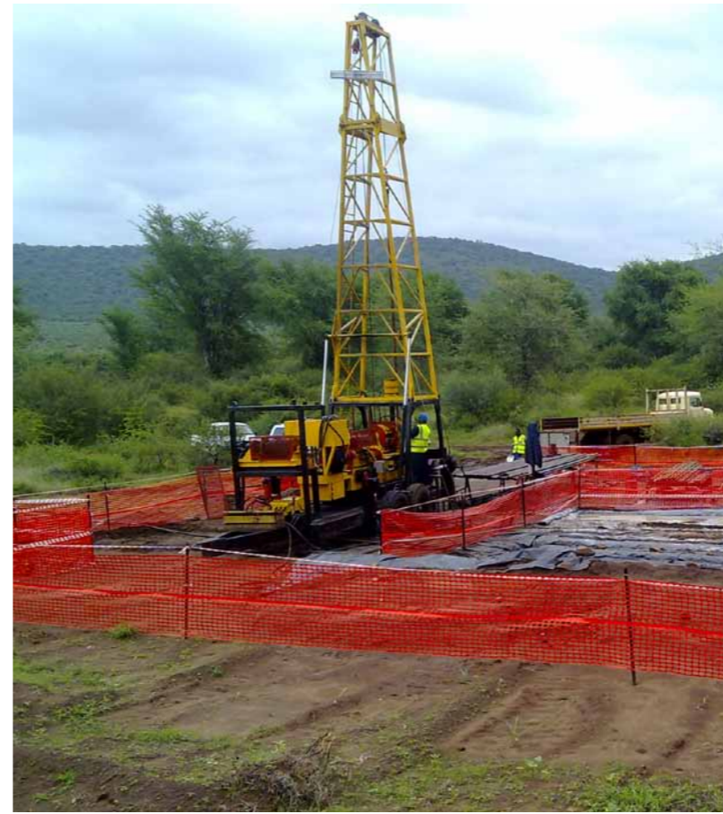
Deep hole drilling at Lesego
