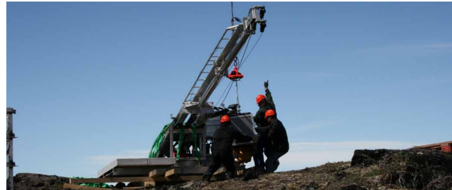
The first drill hole being set up in 2007
