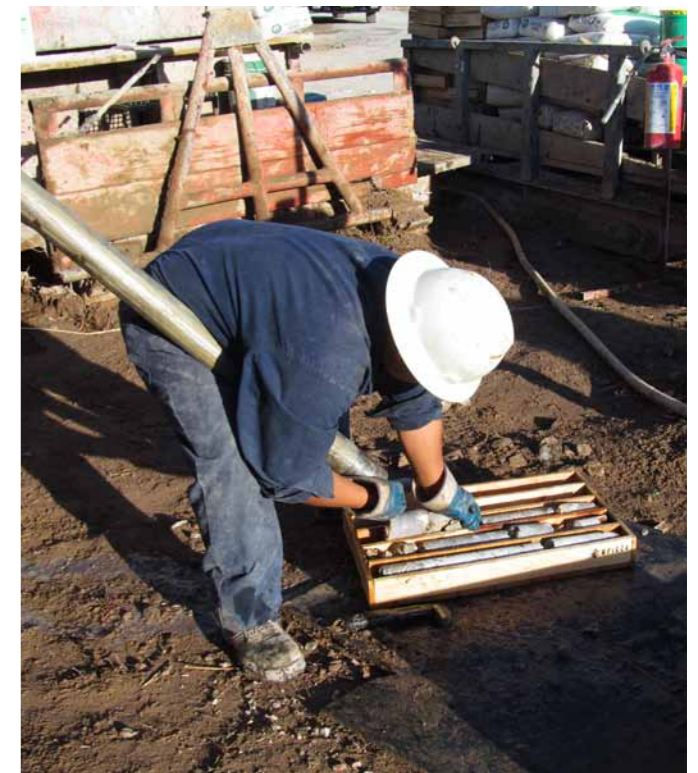
Core removal from the casing
