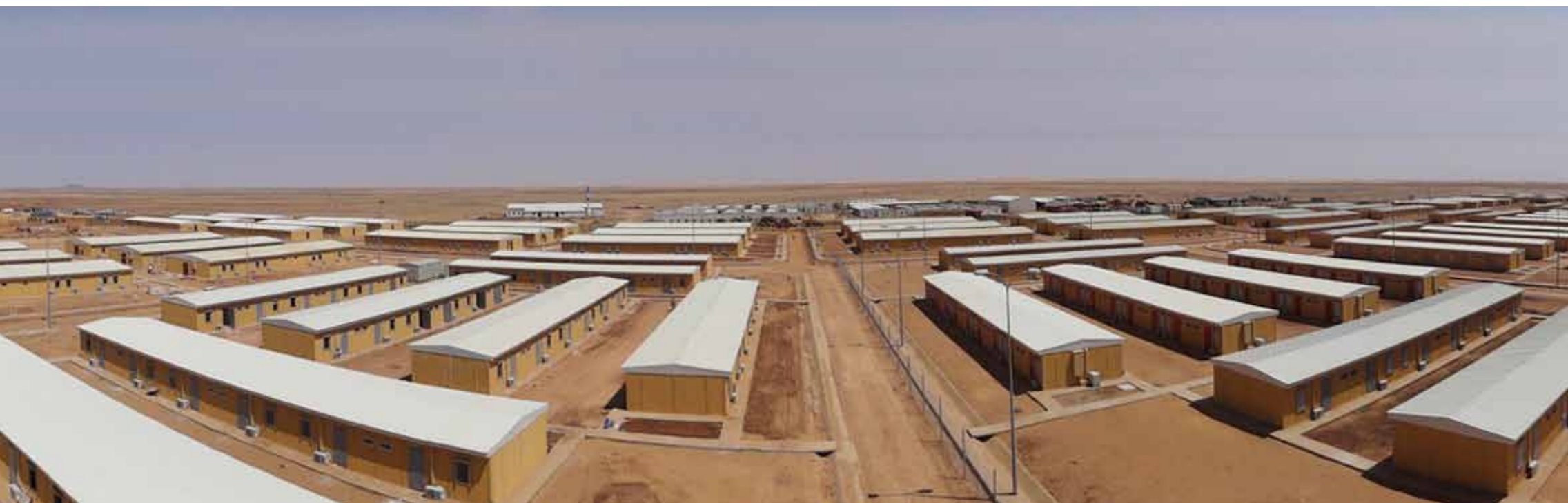
The 8400 person, Tasiast residential village project for mining workers and engineers in Mauritania
