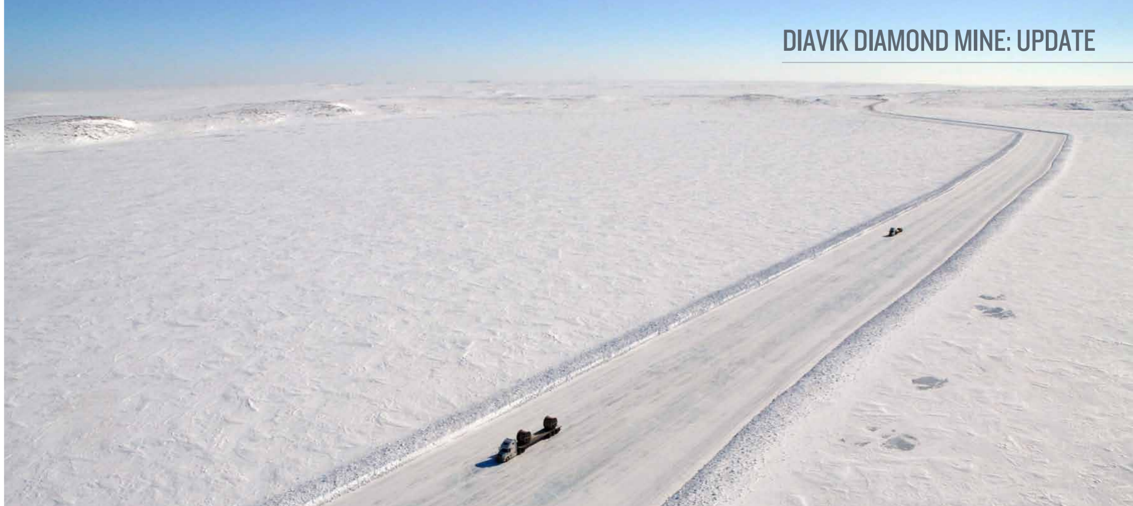
The entire year's supplies of fuel, explosives and cement are brought in on the ice road during its two month operating period
