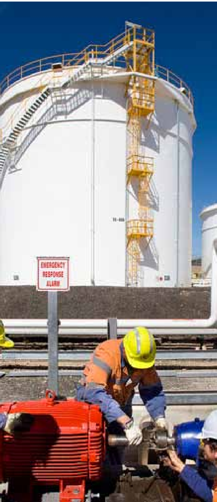
Coogee Chemicals operates bulk liquid terminal facilities
