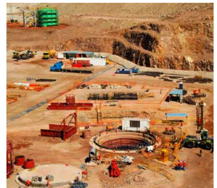
Work platform for air extraction
