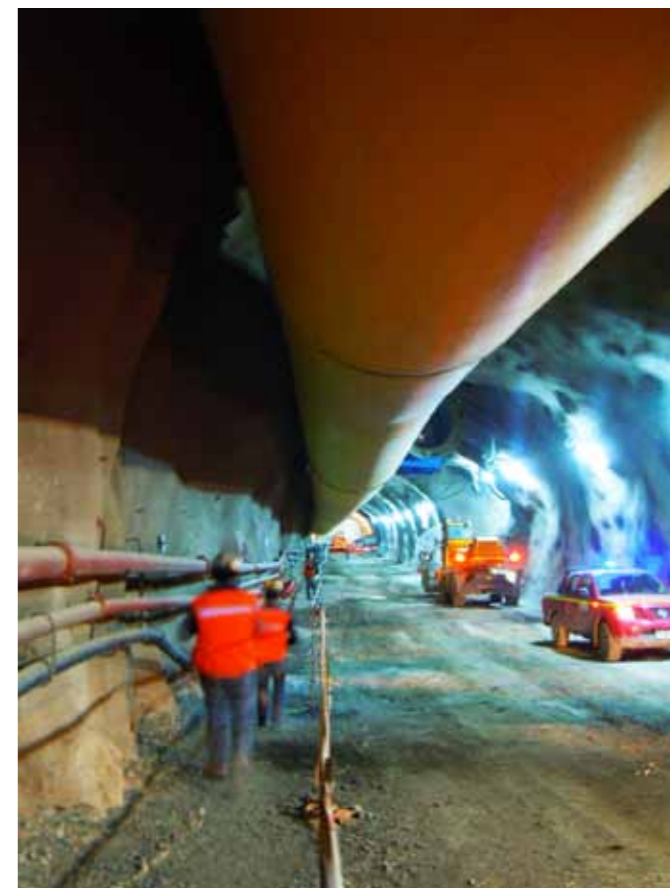
The access tunnel is approximately 7.5km long
