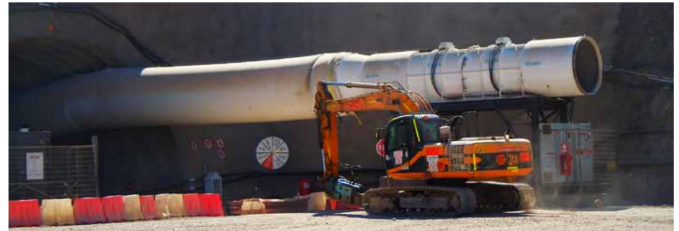
Entrance to tunnel number 12
