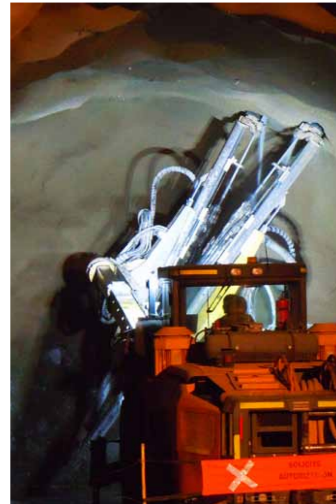
Jumbo rig working in the transport tunnel
