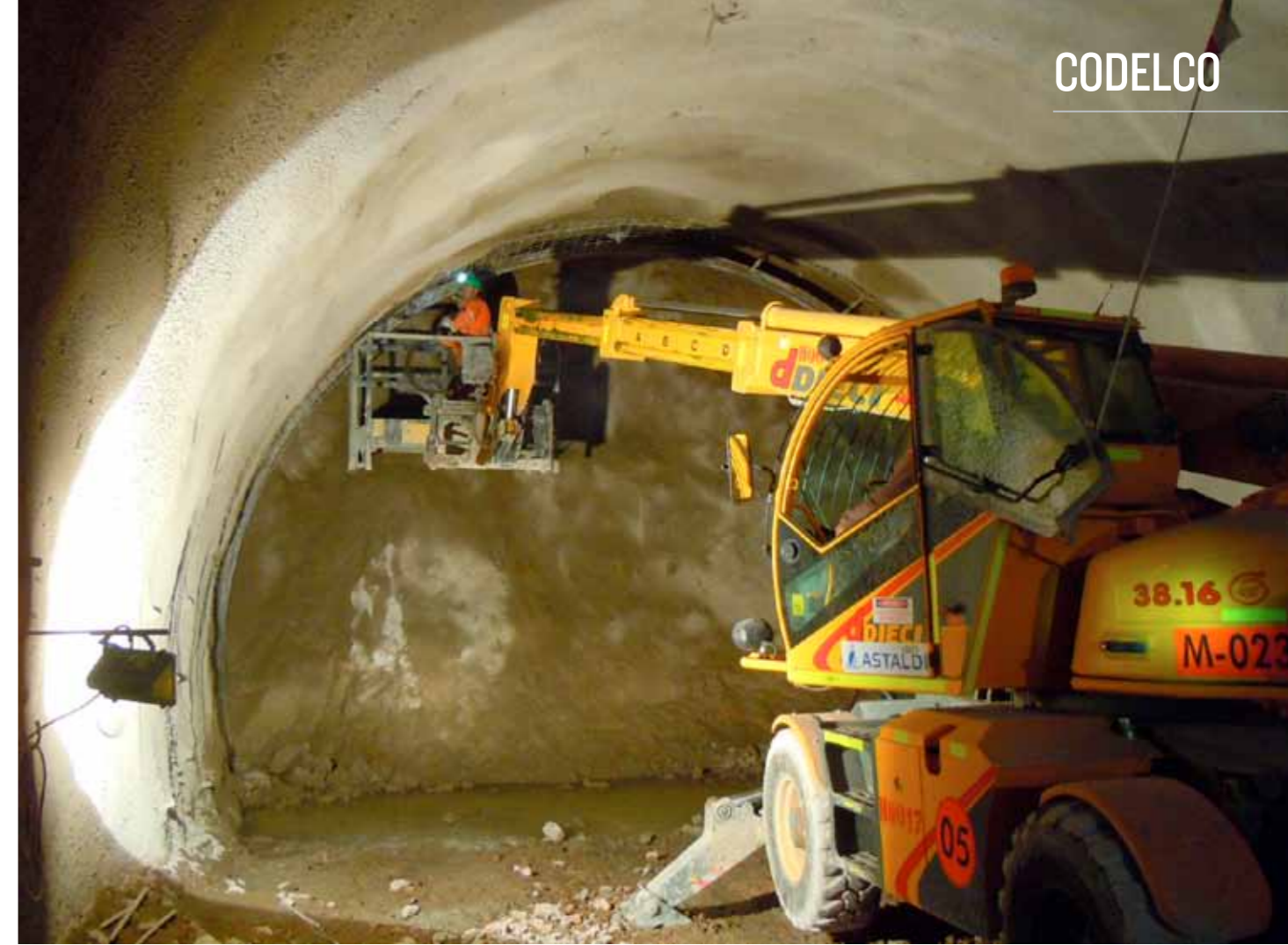
Construction of the underground tunnels at Chuquicamata
