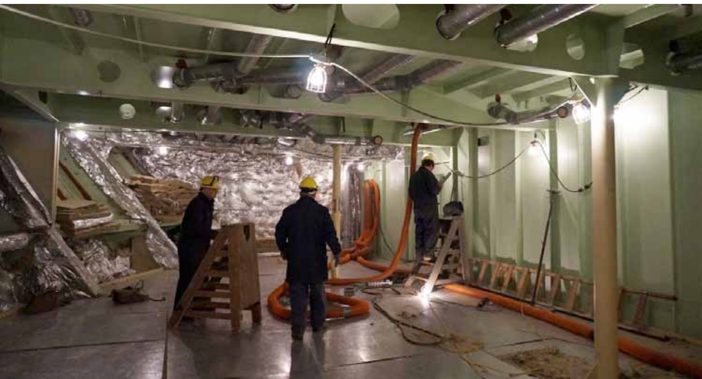
Working below decks
