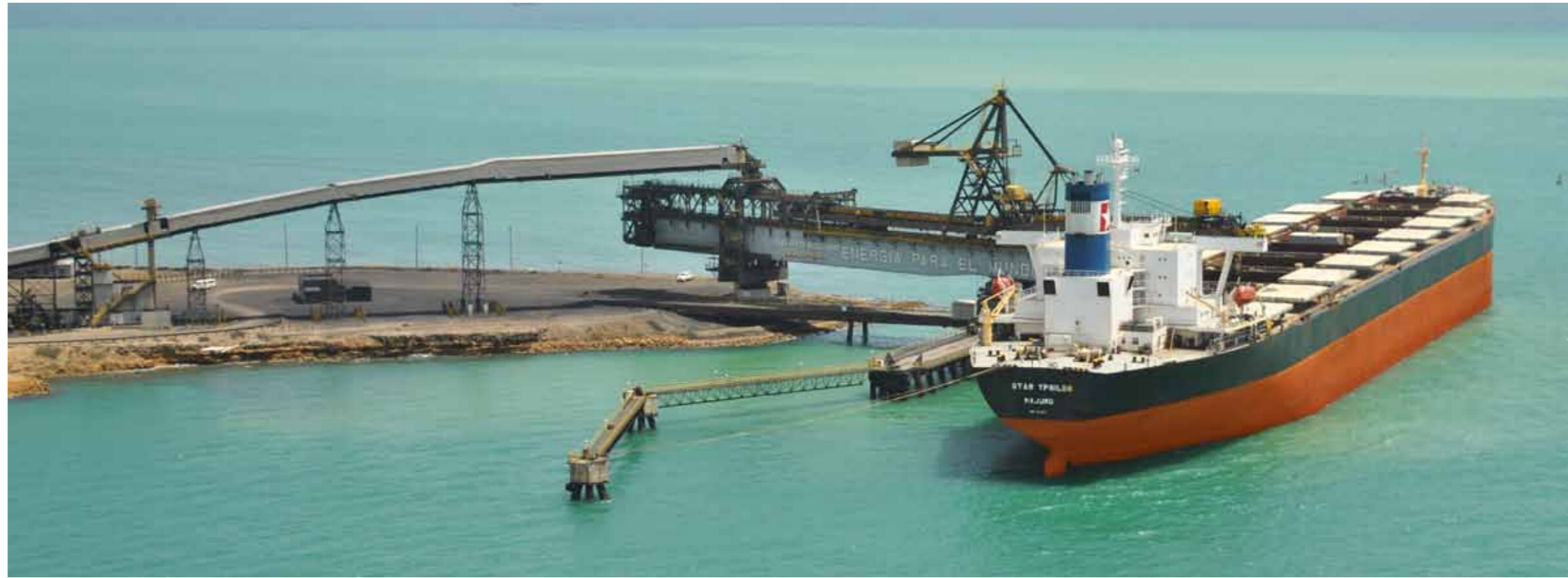
Direct loading of the coal onto the ships, an environmental friendly measure at the port
