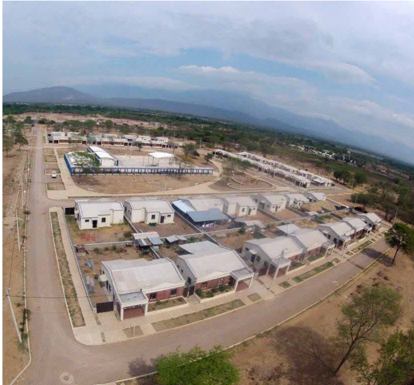
The new site at Chancleta forms part of the resettlement programme
