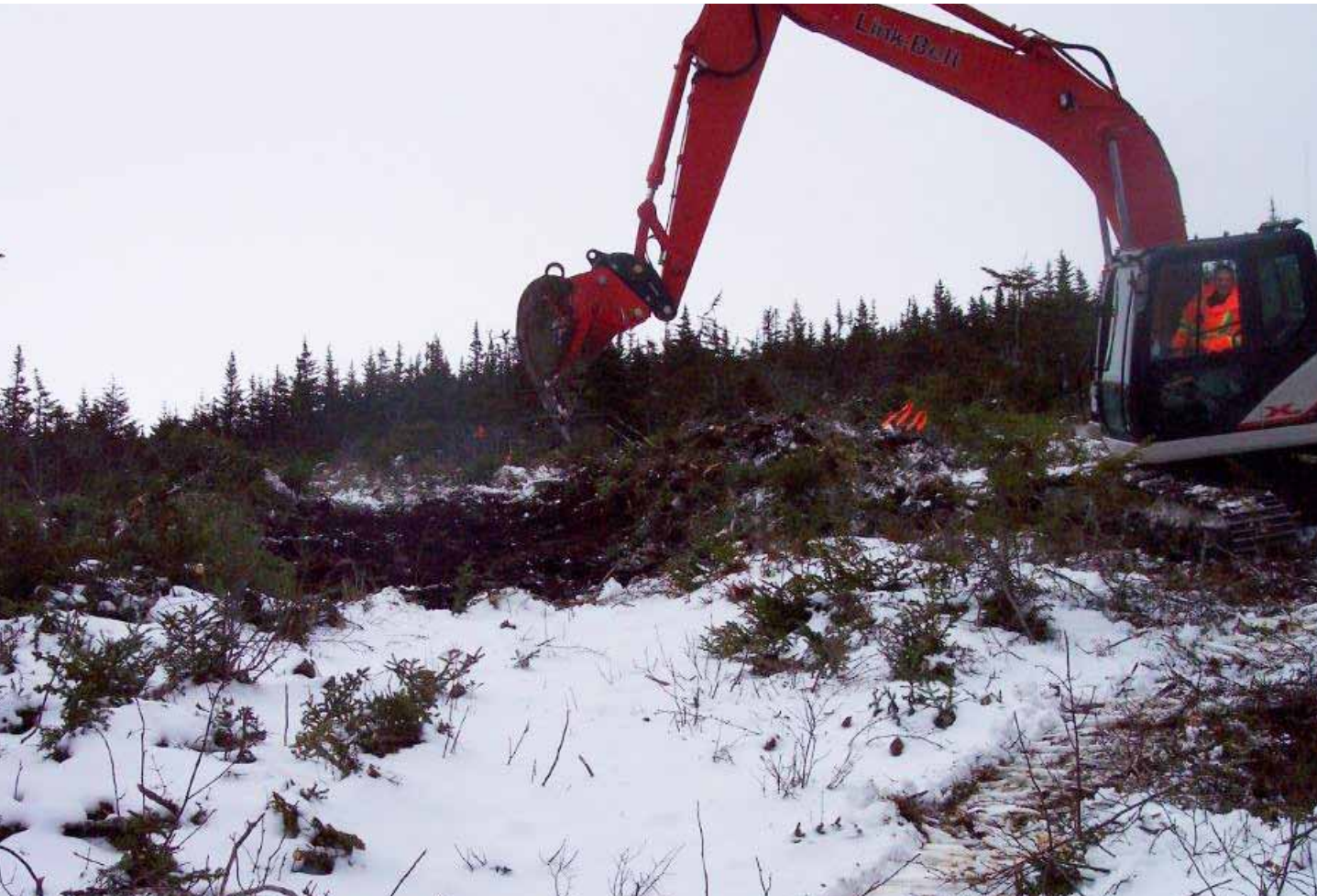
Working in trench two
