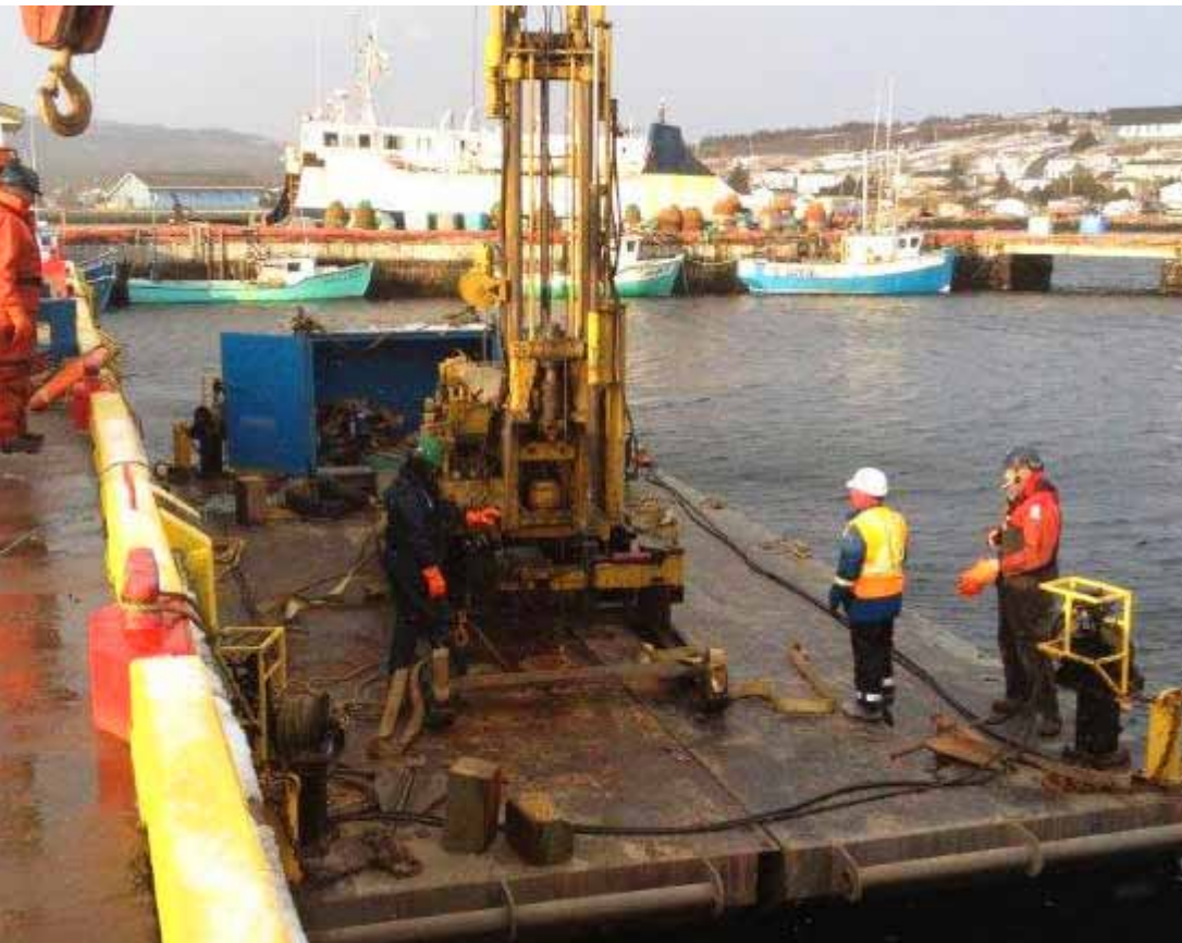
Wharf drilling project
