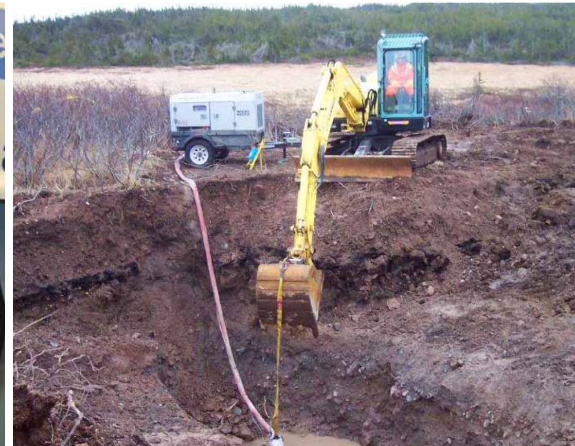
Trenching in the Director vein
