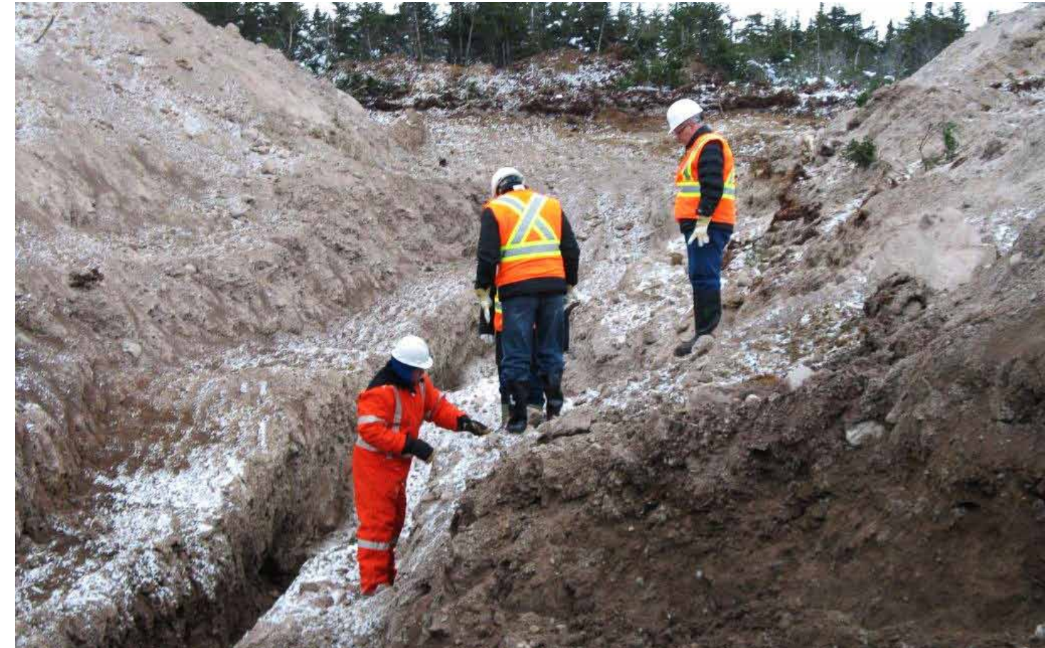
Examining trench three
