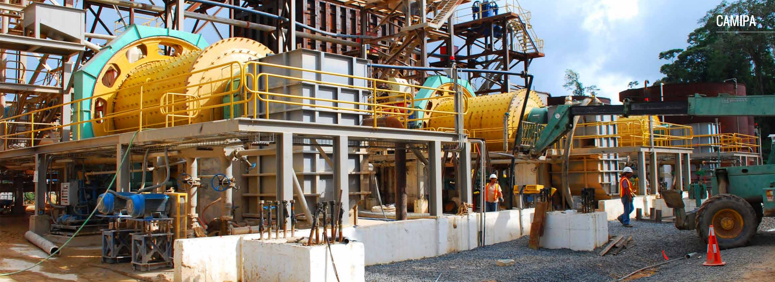
Mills on the Molejón Gold project
